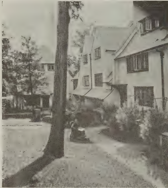
VIEW IN FRONT COURTYARD
